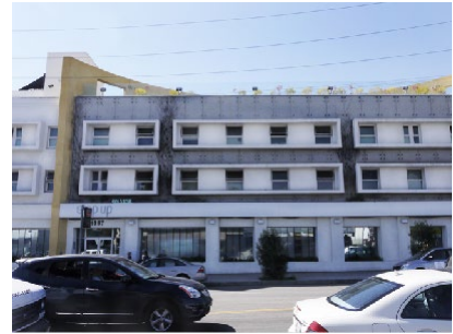
Rehabilitated buildings like Step Up on Vine provide much needed housing and services for the homeless
