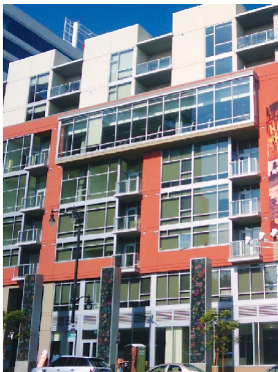
Mixed-use buildings create accessible, walkable, and convenient neighborhoods
